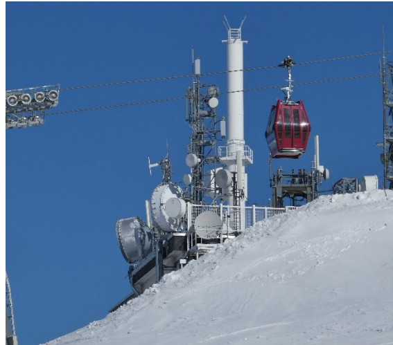
Fig.1. Antennas for microwave links located on the top of the mountain
